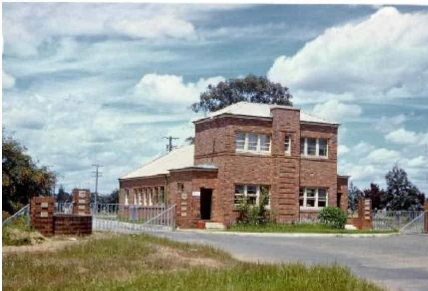
RSTT main entry guard house
